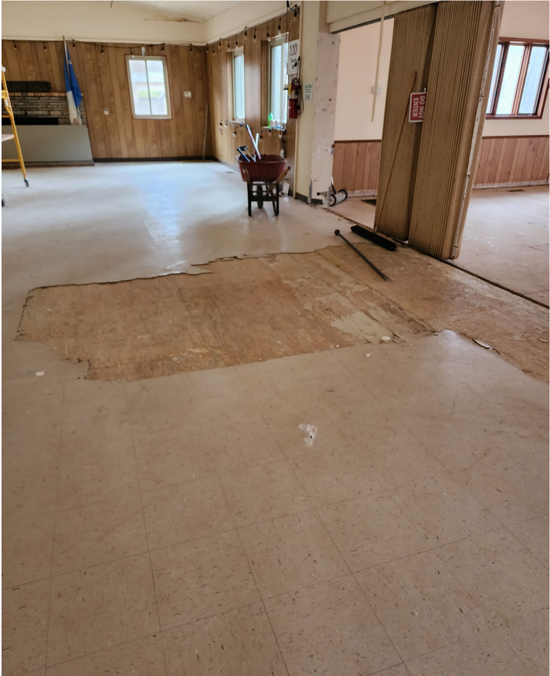
Major Renovation Interior Halsey Dining Hall – Camp Trico (in progress)
