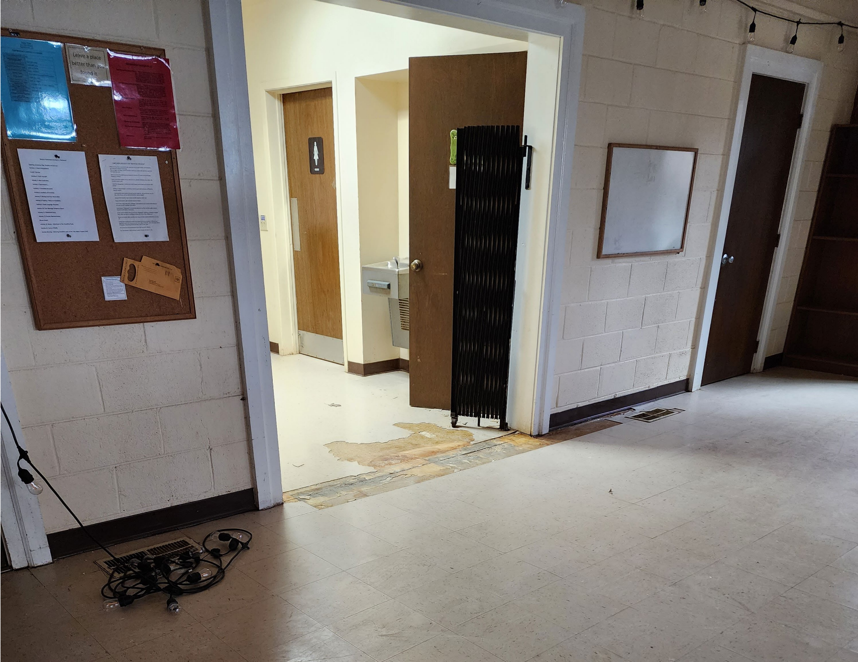
Major Renovation Interior Halsey Dining Hall – Camp Trico (in progress)
