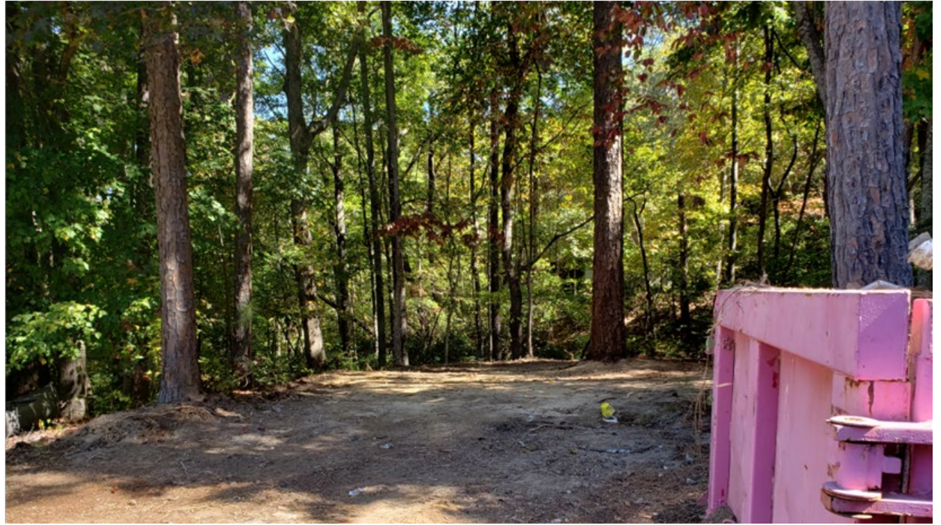
Removal of Octagon Building – Camp Cottaquilla
