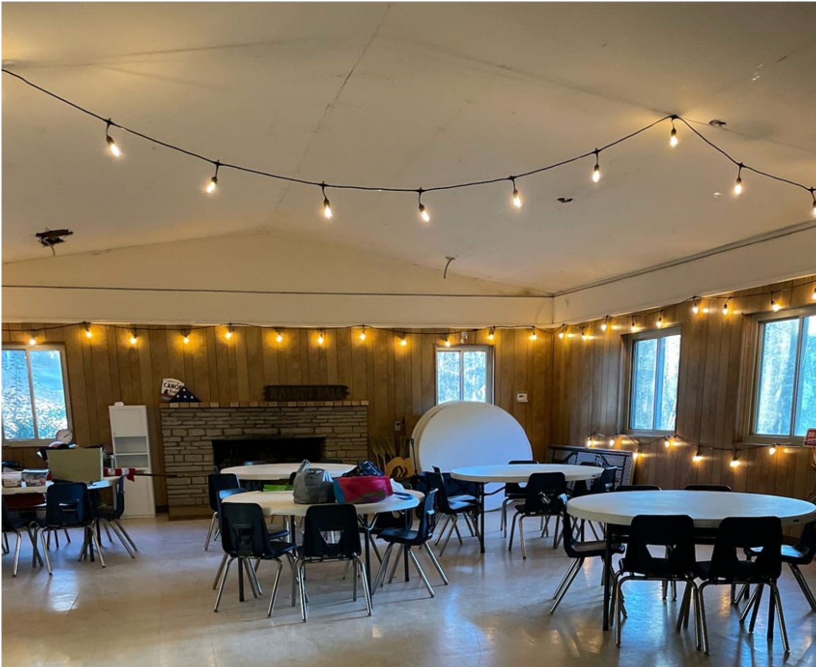
Major Renovation Interior Halsey Dining Hall – Camp Trico (in progress)
